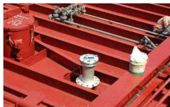
Photos from one of the ships that the JLMD System has been just installed - Sep 2004 Newbuilding launching - S.Korea
